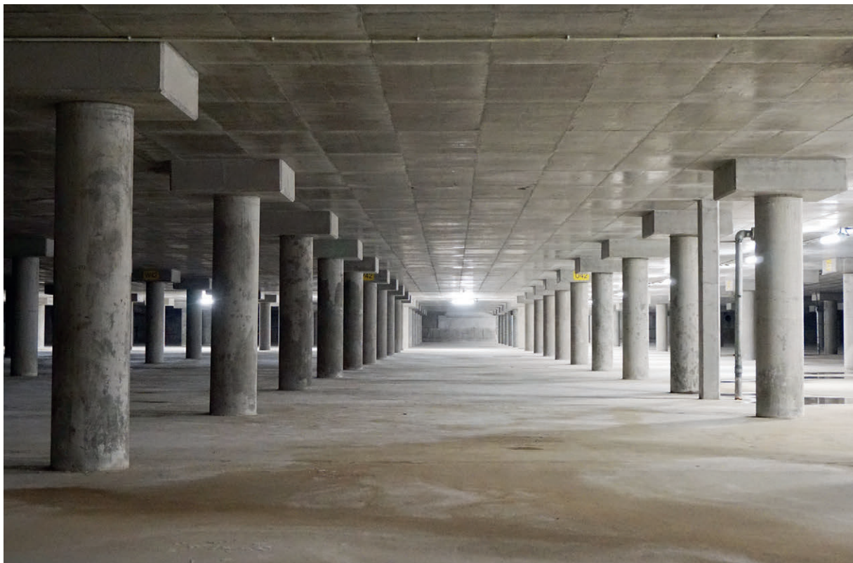
Happy Valley Underground Stormwater Storage Scheme: The stormwater storage tank has a capacity of 60 000 m 3 , which is equivalent to 24 standard swimming pools. It greatly reduces the flood risk to the low-lying areas of Wan Chai and Happy Valley
