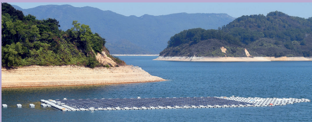
The floating solar energy generation system at Plover Cove Reservoir. The cool and open environment of the reservoir can enhance the efficiency of the solar energy generation system in electricity generation by around 20% as compared with those normally installed on roofs or ground
