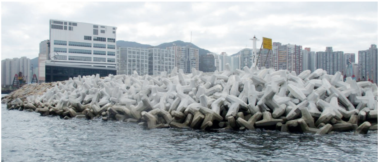
Chai Wan Breakwater
